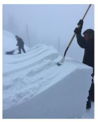
Blowing snow into formwork using a snow blower shown here can help bond and pack the snow so that jumps hold together better throughout the event.
