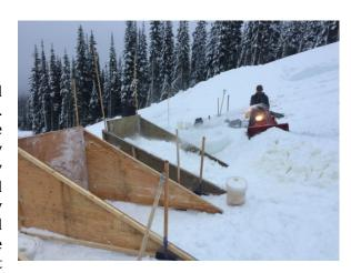
of snowpack, temperatures, skier traffic all go into the decision to add water, Let the jumps set up and consolidate before removing the jump forms.
